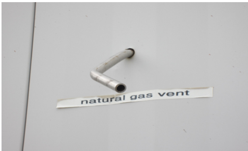
Photo 6. A natural gas vent extruding from the side of an instrument shed at a natural gas well site. The inside diameter of this pipe is about 10 mm (0.25 inch).
