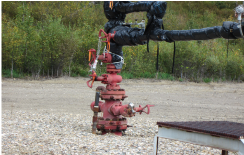
Photo 8. This well (Progress Blueberry C-A39-K/94-a-12) was leaking gas heavily from both the surface-casing vent and the wellhead (middle flange) on August 24, 2016. The well was not operating. It was “shut in”.
