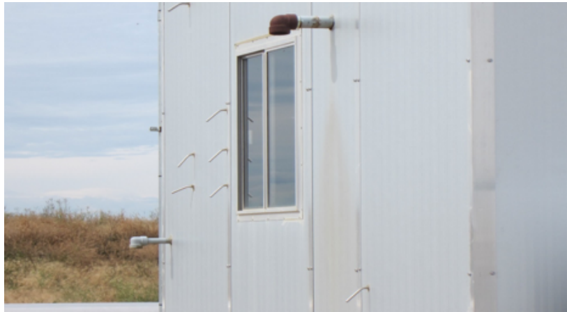
Photo 13. LNG vent pipes extruding from the walls of an instrument shed at well Tourmaline C05-14-18-16 W6M.
